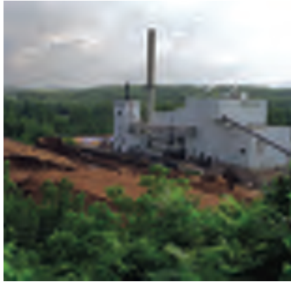
DOE/NREL, PIX 06359, Warren Gretz
